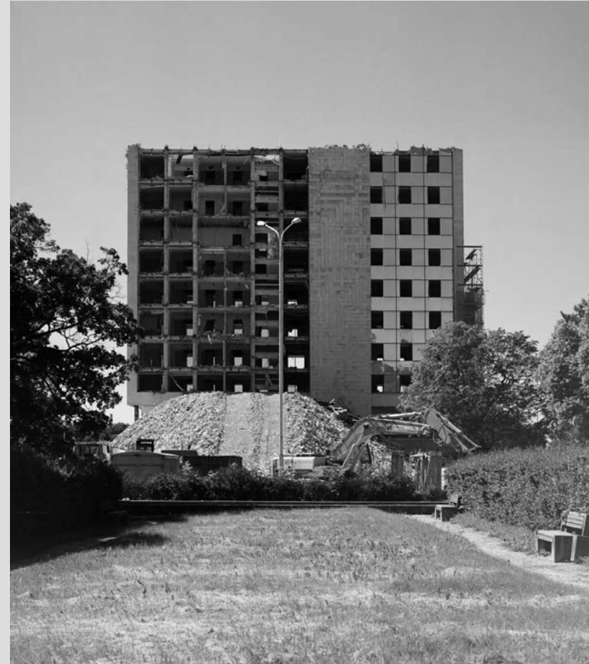
Photo (Tõnu Tunnel): Modernist Tallinn - Buildings from 1970s being demolished
